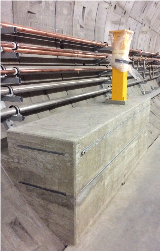
Steel support pillars for 2D-Imager-SR
