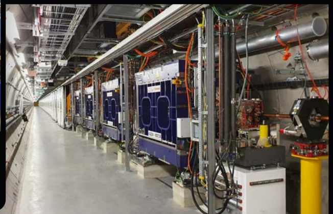
Figure 2: Four new APPLE-X undulator segments installed at the end of the SASE3 undulator
