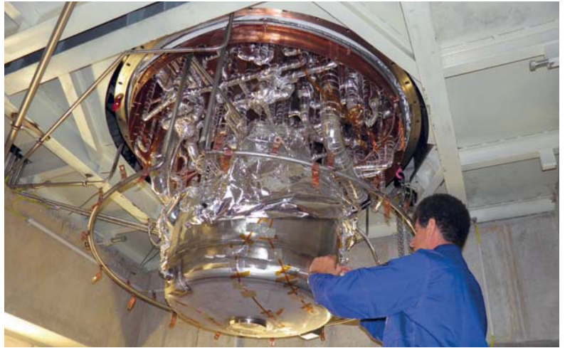
Figure 3 Cryogenic component installed in the first section of the linear accelerator (IKCs DE33 and DE13 by DESY, IKC RU24 by BINP)
