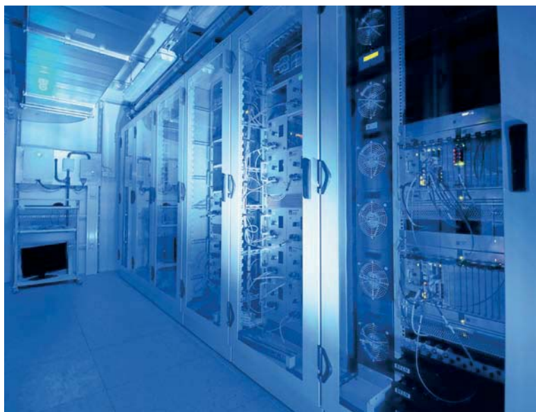
Figure 1 Electrical infrastructure room for the FXE instrument including complex control electronics, such as high-speed electronics (front) and PLC modules (back)
