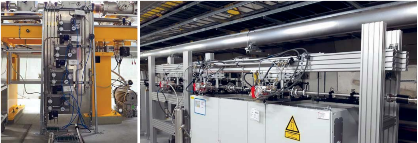
Figure 2 Infrastructure for gas-based online diagnostics. Left Gas panel in XTD2 at the XGM. Right Hanging differential pumping stage in SASE3.
