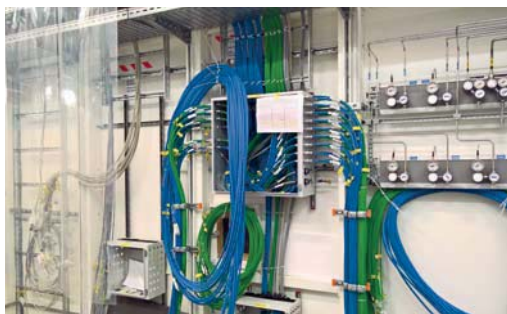
Figure 3 Motor and encoder cables installed in the SPB/SFX instrument
