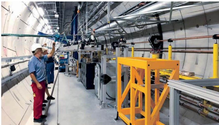
Figure 3 Installation of a differential pumping system in XTD1 with the help of the DESY Hall Service and Transport group. The electron beamline is already installed on the right side of the tunnel.
