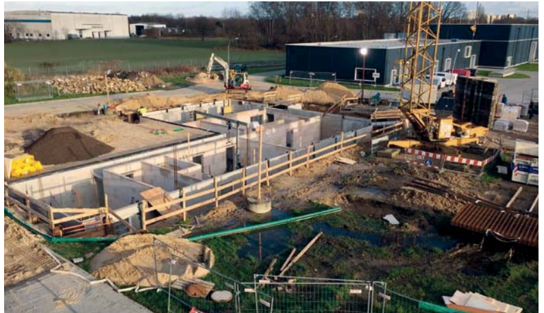
Figure 4 Civil construction site for the canteen building (XHC) in December 2017
