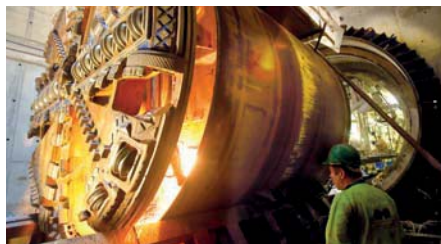
Figure 10 First tunnel boring machine after its arrival in the final shaft
