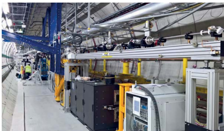
Figure 1 Electron beamline (right) and photon beamline (left) in the tunnel XTD1 looking downstream. The large blue steel structure provides support for the very sensitive X-ray gas monitor. The electron beamline is complete, and final installation activities are taking place on the photon beamline.
