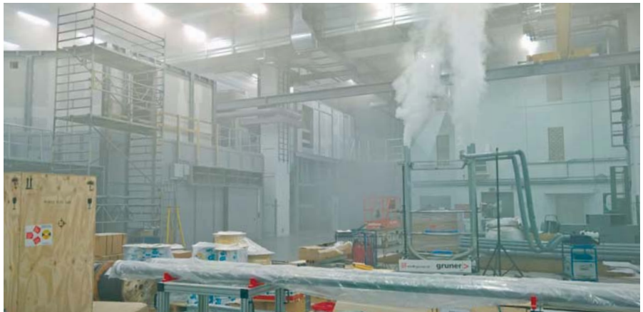
Figure 2 Test of the smoke extraction system in the experiment hall performed by introducing special artificial smoke
