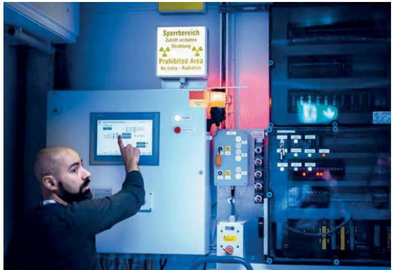
Figure 8 Personnel interlock (DE38 by DESY)
