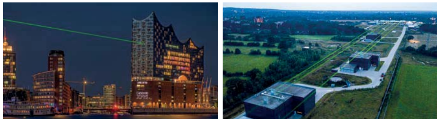
Figure 17 Laser installation from the Elbphilharmonie in Hamburg (left) and from roof of the European XFEL main building in Schenefeld (right). Hamburg says 'welcome' to European XFEL, and the facility sends five laser beams highlighting the underground tunnels to Hamburg.
