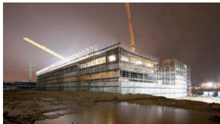
Figure 12 The European XFEL headquarters building (XHQ) under construction in December 2014
