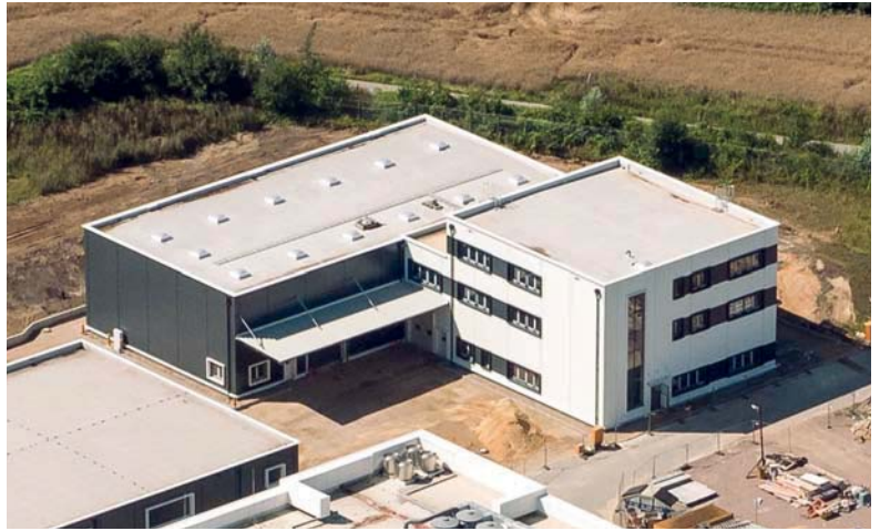
Figure 3 Workshop and storage building (XHWS) in August 2017
