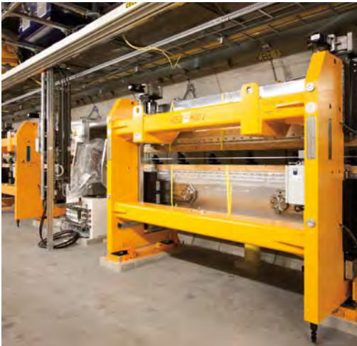
Figure 3 Undulator segments installed in the XTD2 tunnel
