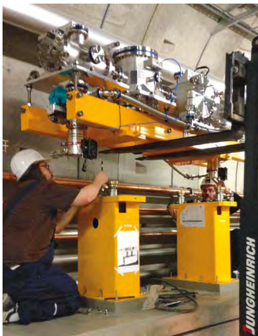
Figure 1 First tunnel installation of an XGM (November 2015)
