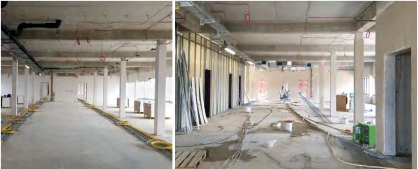
Figure 6 Views of the second floor of XHQ (September 2015)
