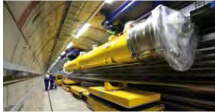
Figure 17 Installation of the first completed and tested accelerator module in the tunnel in August 2014
