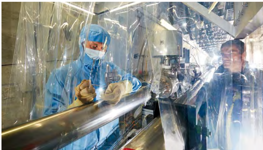
Figure 2 Installation work in the XTD9 tunnel. To avoid particle contamination of the sensitive X-ray mirrors, the beam pipes and vacuum chambers are being connected using mobile cleanrooms.
