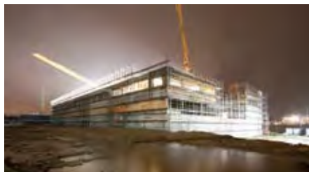
Figure 16 The European XFEL headquarters building (XHQ) under construction in December 2014
