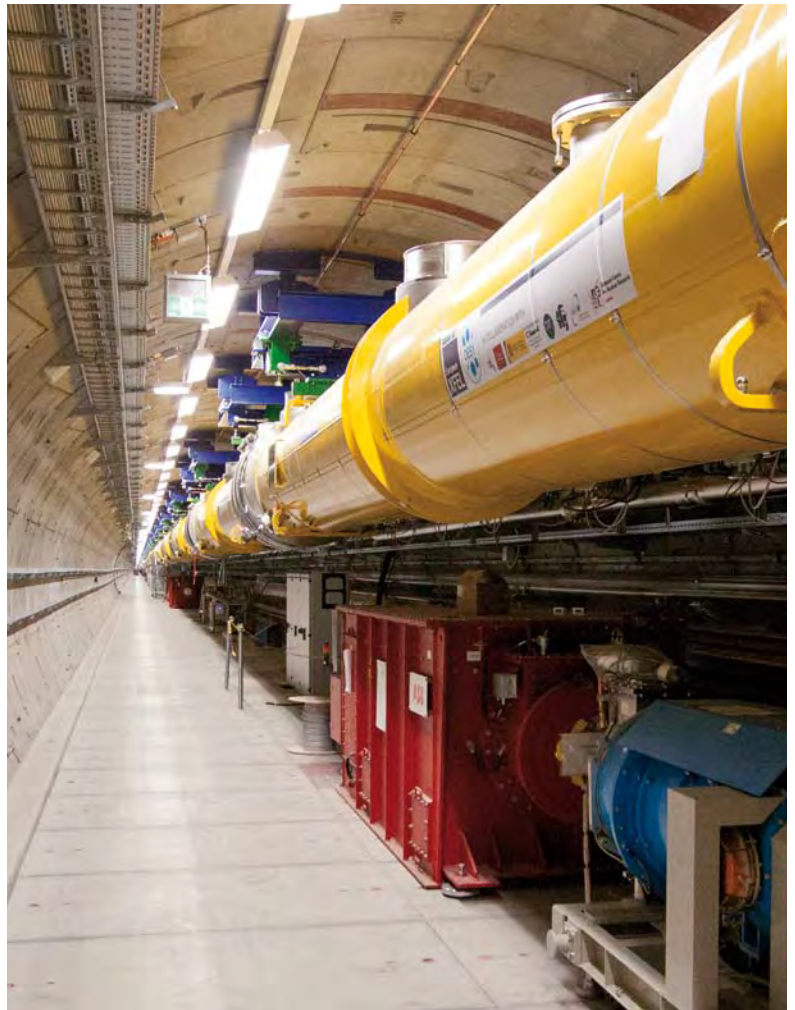
Figure 4 Cryomodules assembled (IKC FR03 by CEA) and installed in the tunnel (IKC DE33 by DESY)
