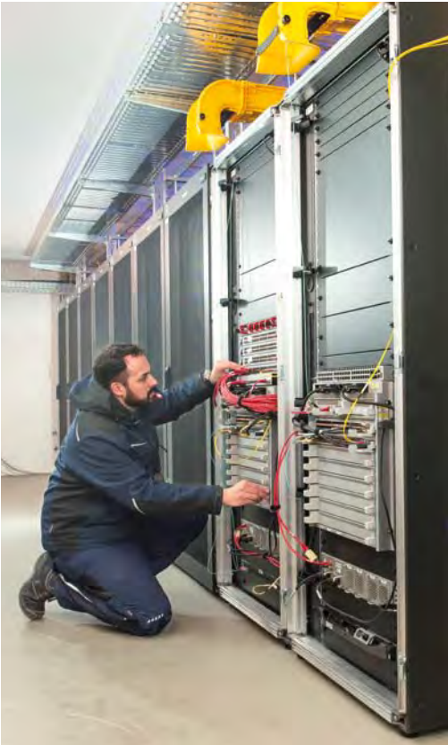
Figure 1 Installations in the balcony rooms of the experiment hall
