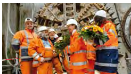
Figure 14 Arrival of the second tunnel boring machine in the final reception shaft on 4 June 2012
