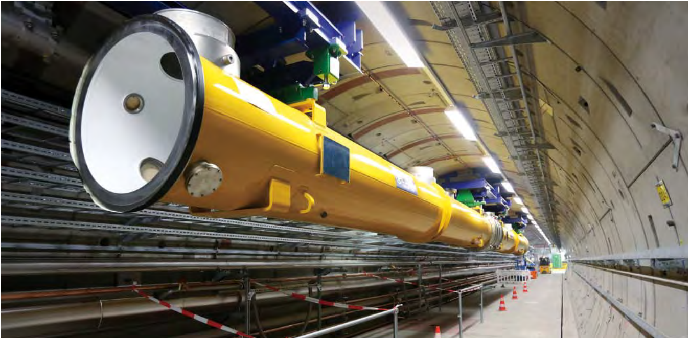
Figure 1 Cryostat delivery (42 from IKC IT02/WP03 by INFN) and installation (IKC DE33 by DESY). The delivery of the remaining cryostats will be managed by WP03 and in particular through IKC DE03 by DESY.
