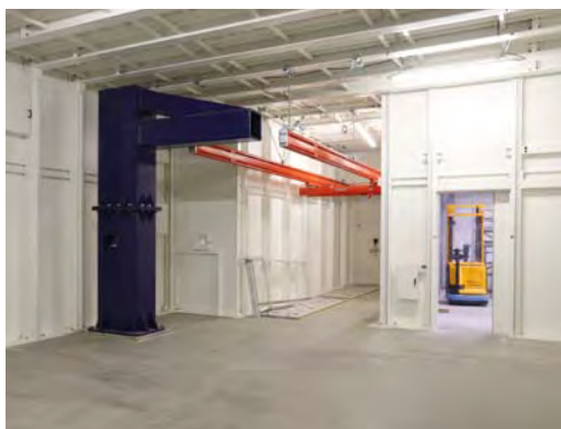
Figure 2 FXE robot tower installed inside the experiment hutch
