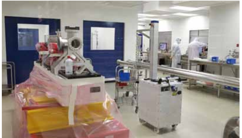
Figure 5 Installation of vacuum components on girders in the cleanroom (August 2014)
