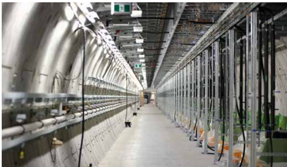
Figure 1 View of XTD2 with support structures for the undulators
