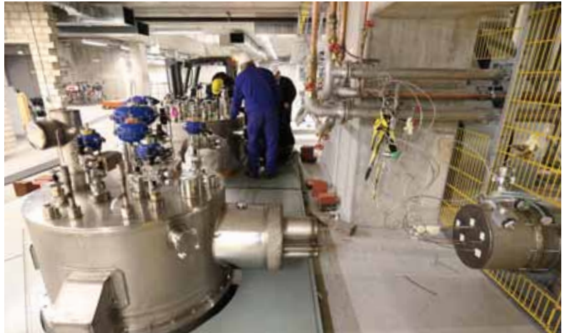
Figure 6 Installation of the cryo-valve boxes for the injector and linear accelerator cryogenic supply (November 2014)
