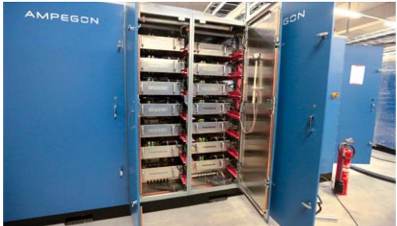
**Figure 3** View into one of the first power modulators supplying the klystrons in the accelerator tunnel of the European XFEL
