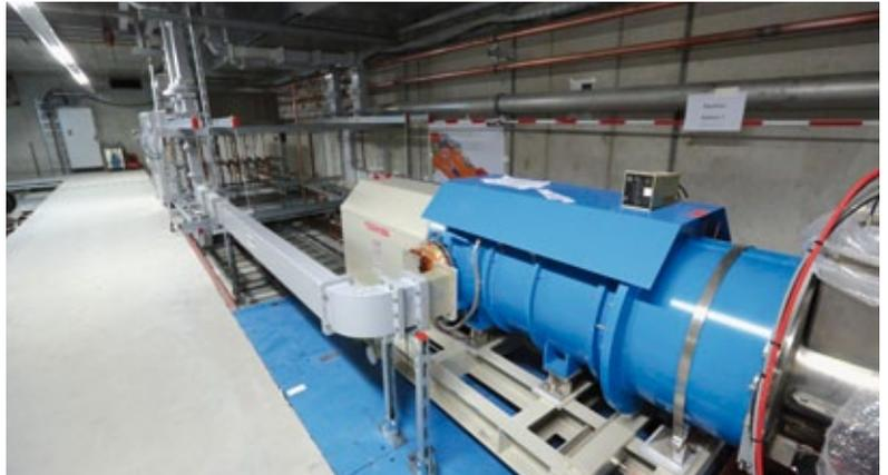
**Figure 5** First multibeam klystron installed in the XTIN underground building. The klystron supplies RF power to the RF gun installed in the injector tunnel. The connection is done using rectangular waveguides.
