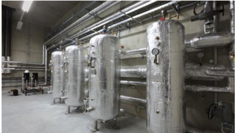
**Figure 7** Hot-water reservoirs for gun temperature control installed on the seventh floor of XTIN
