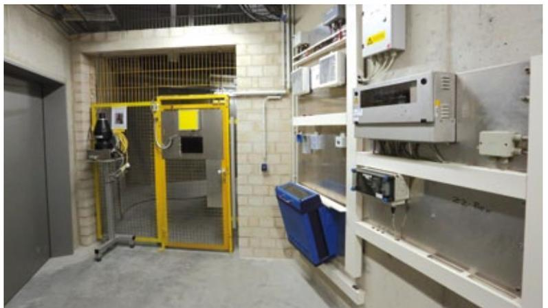
**Figure 8** Interlock door from XSIN to XTIN with a temporary-access key system and radiation-monitoring device
