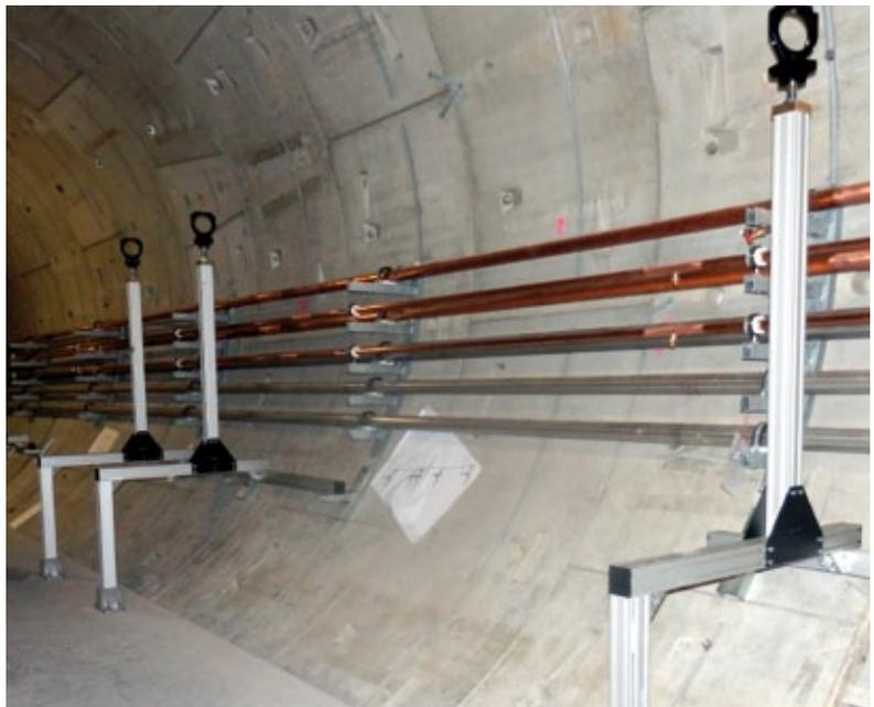
**Figure 3** First installation of beam pipe supports in XTD2. The X-ray beam will be located on top of the aluminium structure, where UHV beam pipes will be installed.
