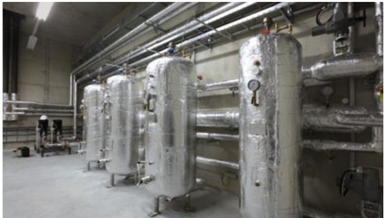
**Figure 7** Hot-water reservoirs for gun temperature control installed on the seventh floor of XTIN
