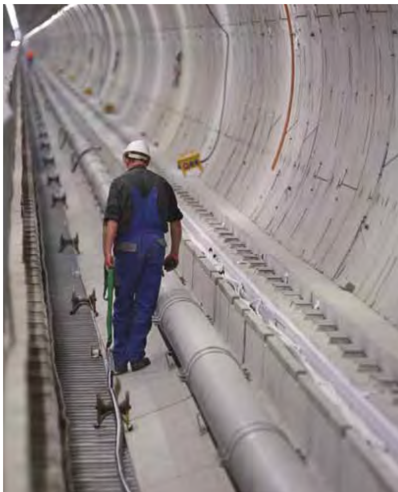
Figure 9 Installation of a pulse cable in the open space beneath the tunnel floor
