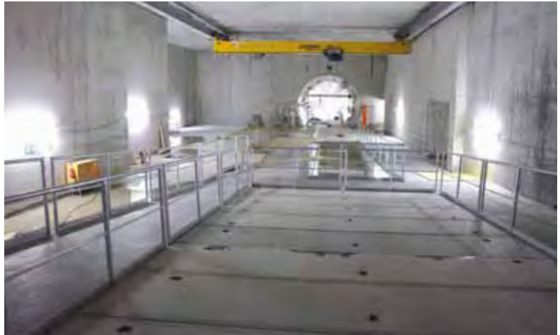
Figure 10 View into the accelerator tunnel XTL from inside the shaft building XS1 (November 2012)
