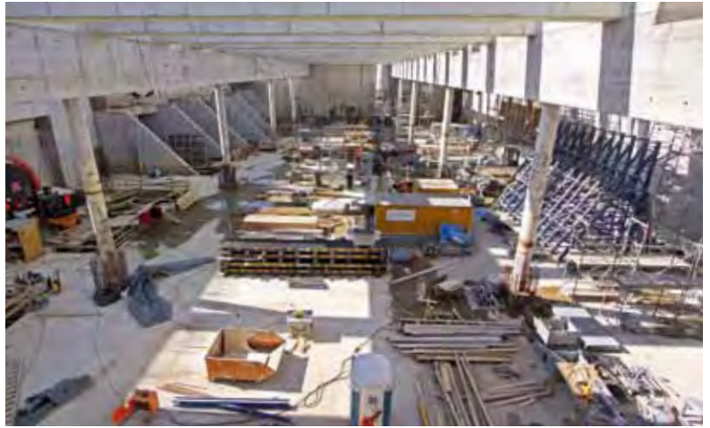
Figure 13 Work in the experiment hall XHEXP1 (April 2012)
