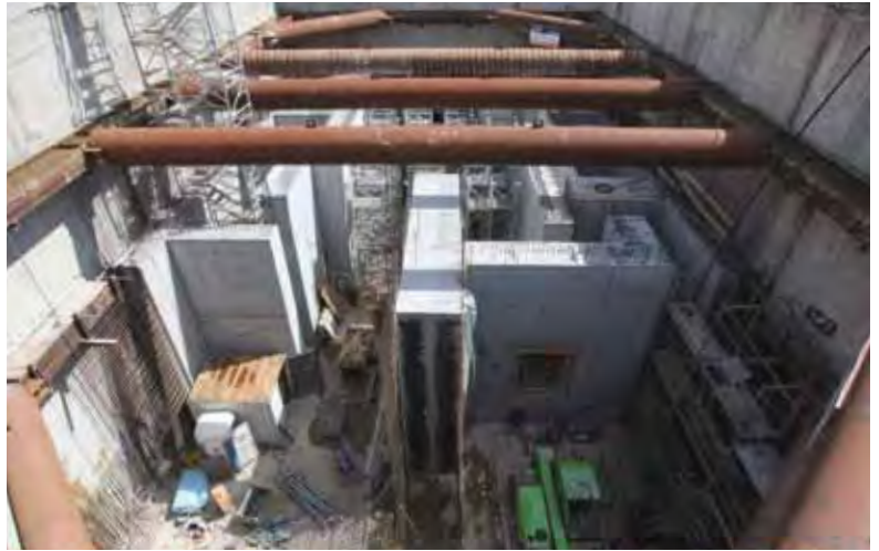
Figure 11 Civil construction work inside the shaft XS3 (August 2012)
