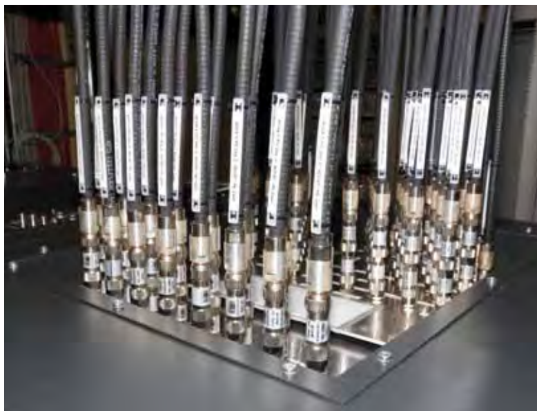
Figure 5 Patch panel connecting the RF signal cables to the LLRF system
