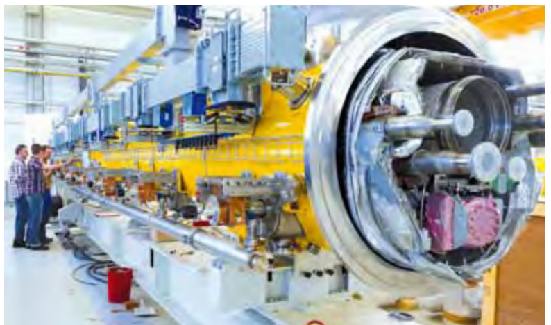
Figure 4 Prototype accelerator module fully assembled with auxiliary equipment like waveguides, cable tray, and coupler vacuum pipes
