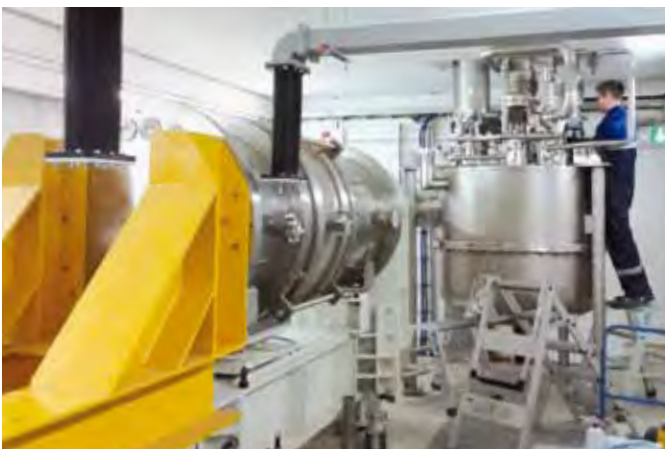
Figure 9 Contract to BINP: Assembly of cryogenic equipment for accelerator module test bench
