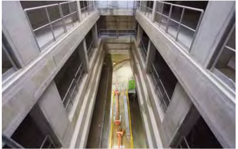
Figure 7 View into the entrance shaft of the injector complex XSE (August 2012)
