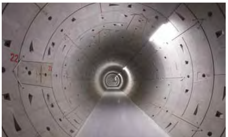
Figure 5 View into the completed tunnel XTD3 (November 2012)
