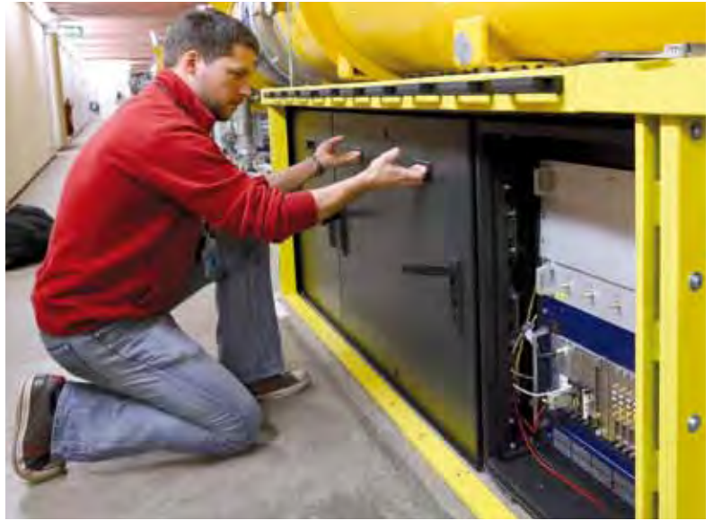
Figure 7 LLRF electronics installed in a shielded rack underneath an accelerator module in the FLASH facility. The installation is similar to the situation in the European XFEL injector. In the linear accelerator tunnel, the LLRF racks will be higher.
