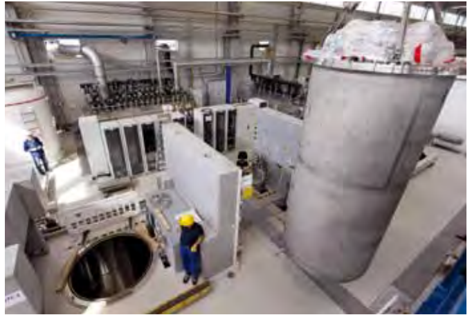
Figure 8 IKC by WUT: Installation in AMTF of a vertical cryostat for testing superconducting cavities
