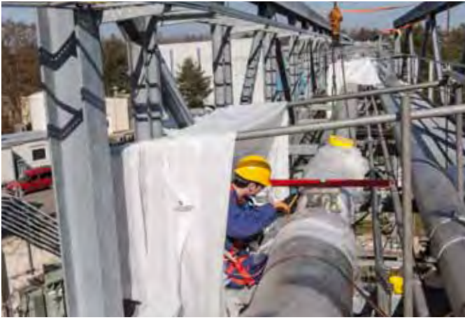
Figure 7 IKC by WUT: Production and installation of a 150 m long helium transfer line
