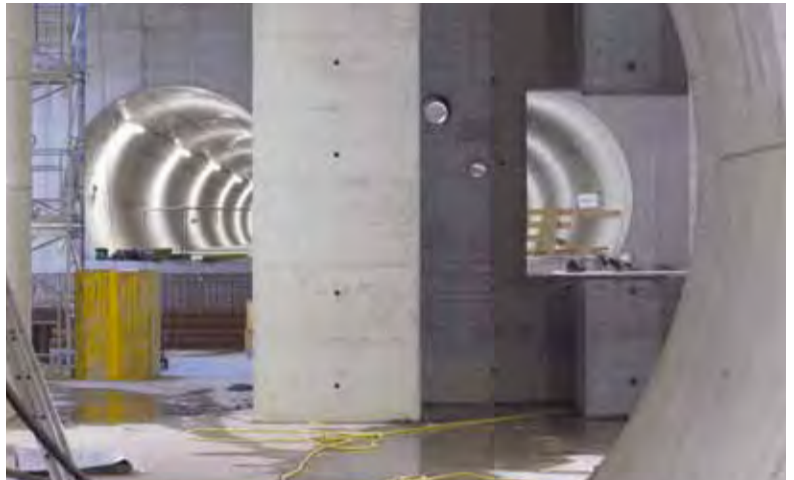
Figure 12 View from the tunnel XTD3 through the shaft XS4 into the tunnels XTD5 (left) and XTD8 (right) in November 2012
