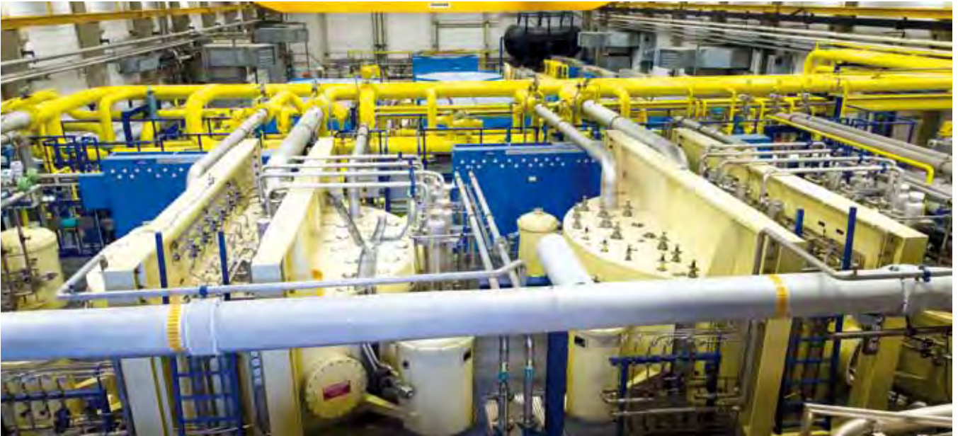
Figure 7 The former DESY HERA refrigeration plant is being remodeled and modernized for the European XFEL.
