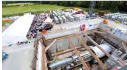
Figure 12 First tunnel and borer christening ceremony on the European XFEL construction site Schenefeld on 30 June 2010
