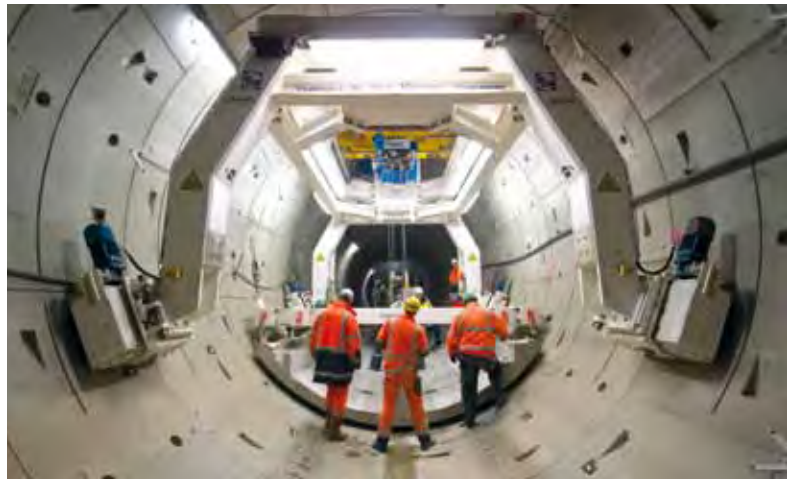
Figure 7 Floor construction in the linear accelerator tunnel
