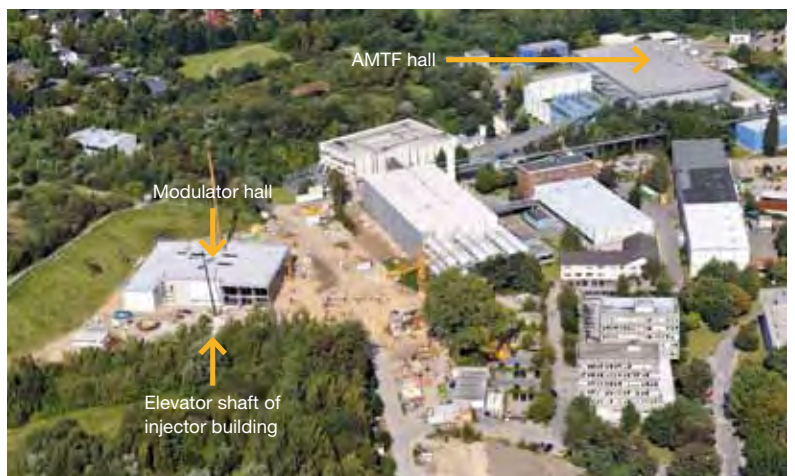
Figure 9 Aerial view of the injector complex region (September 2011)
