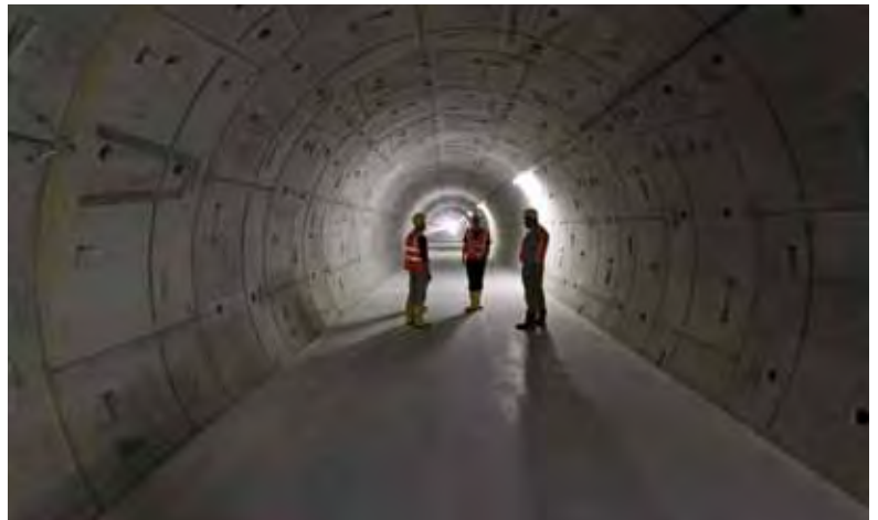
Figure 8 Floor construction of the first undulator tunnel
