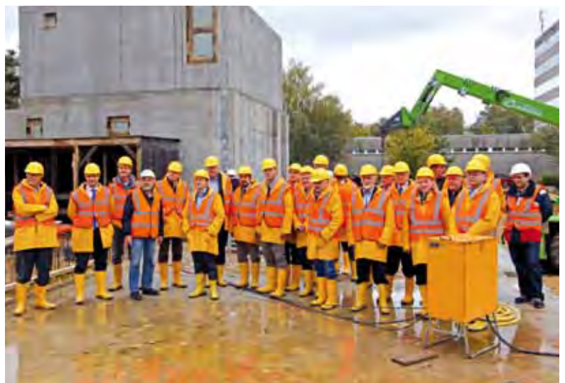
Figure 1 Accelerator Consortium Board during a visit to the European XFEL construction site
