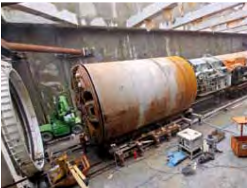
Figure 3 TULA being moved into its starting position in Shaft 1 (January 2011)
